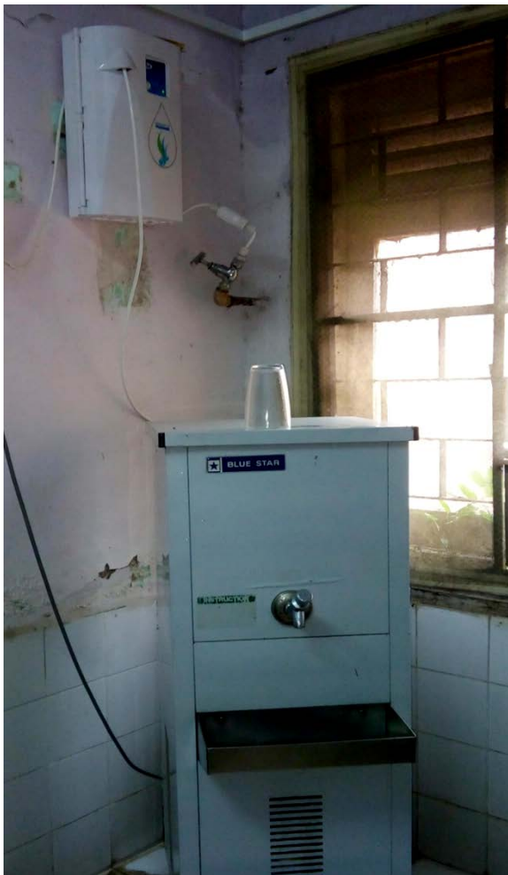
Water Cooler along with Water Purifier
